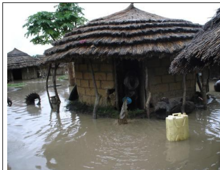
Figure 36: Flooded rural home in Eastern Uganda
